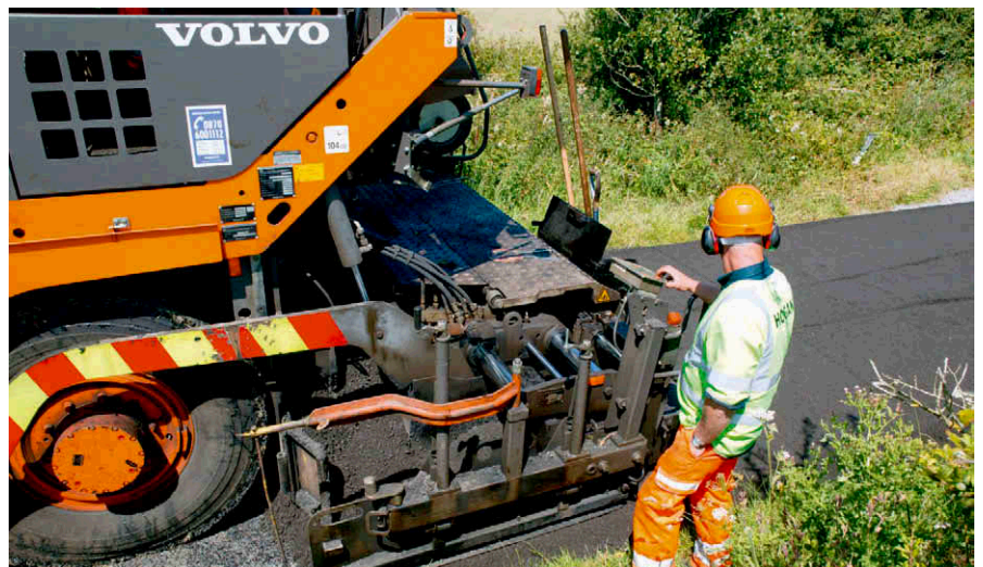
Asphalt material laid on three sites in North Wales contained no virgin aggregates
