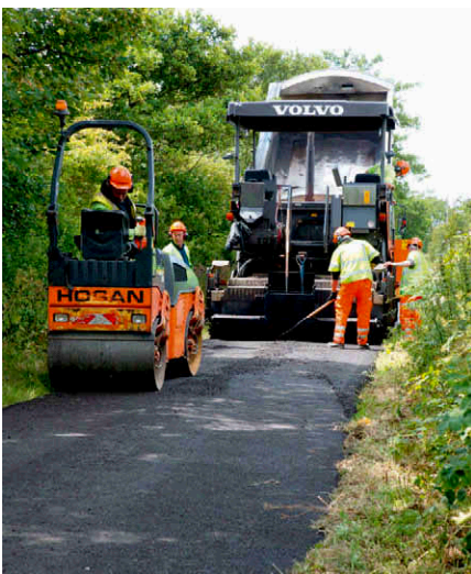
Asphalt material laid on three sites in North Wales contained no virgin aggregates
