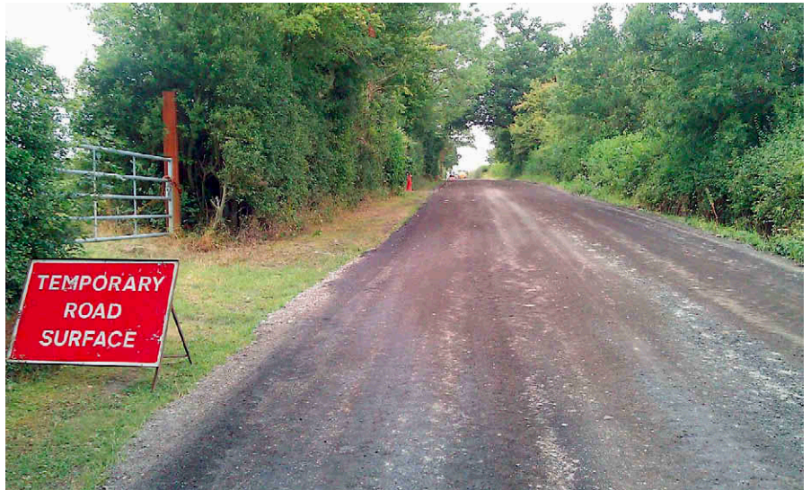
In situ recycling represents a cost effective means of renewing worn carriageway
