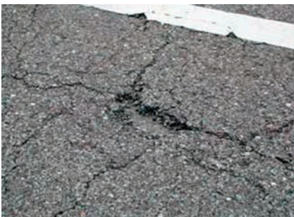
Results from the Lausanne study of binder performance, particularly 'cracking index' results, showed great variation between different polymer modified binders. Some PMB binders (above left) performed poorly in comparison to standard penetration grades. The Styrelf section is shown above right
