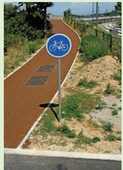
Shell Floraphalte: the clear binder mixed with pigment produces long lasting colour
