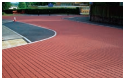
Recent uses of the StreetPrint process include residential works in Wiltshire
