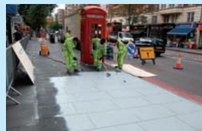
An even and aesthetic footway surface has been created beside the Edgware Road using StreetPrint 150 finished with an off-white colouring
