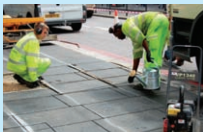
An even and aesthetic footway surface has been created beside the Edgware Road using StreetPrint 150 finished with an off-white colouring
