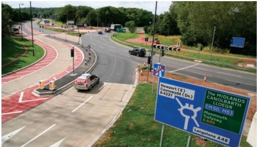
High friction surfacing can perform well for long periods – if applied correctly
