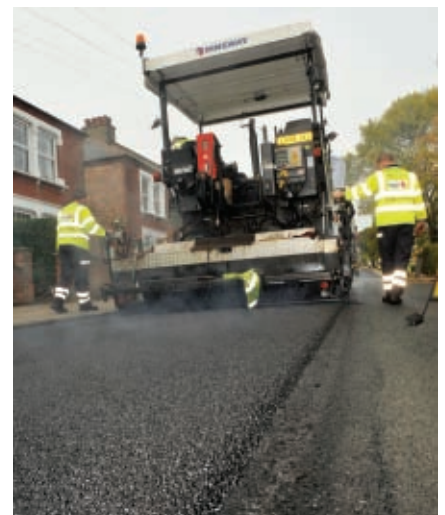
Road renewal under way in Enfield, north London
