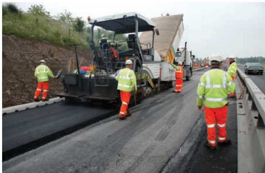
Major schemes have been carried out in recent months using PMBs in surface and base layers
