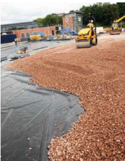
TarmacDry features carefully chosen aggregates over an impermeable membrane plus surfacing with porous asphalt to handle very high volumes of water
