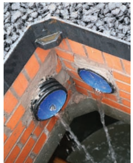
TarmacDry features carefully chosen aggregates over an impermeable membrane plus surfacing with porous asphalt to handle very high volumes of water
