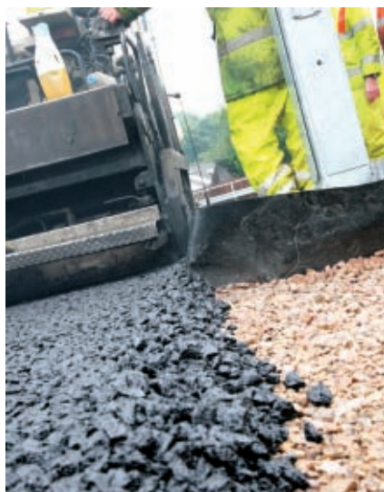
TarmacDry features carefully chosen aggregates over an impermeable membrane plus surfacing with porous asphalt to handle very high volumes of water
