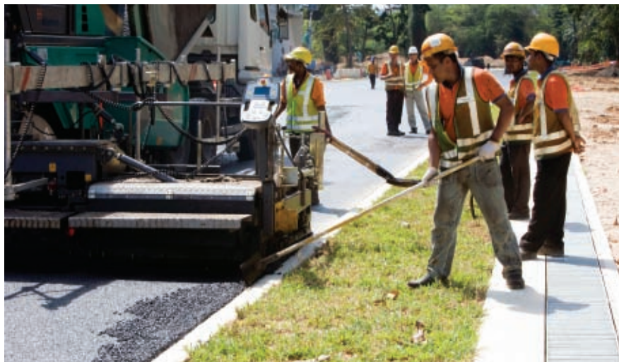
Shell Bitumen's Cariphalte Racetrack binder has a high cohesive strength for withstanding high forces
