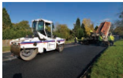
A roller compacted Ultraphone to a depth of 60mm
