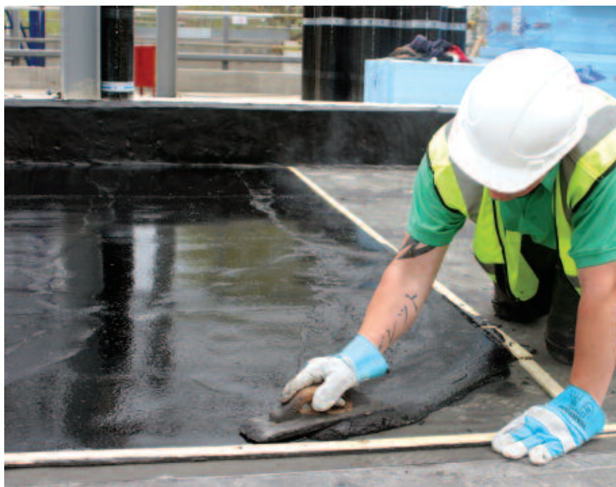
Using Shell S Grade binders has many benefits including reducing energy costs and emission of fumes
