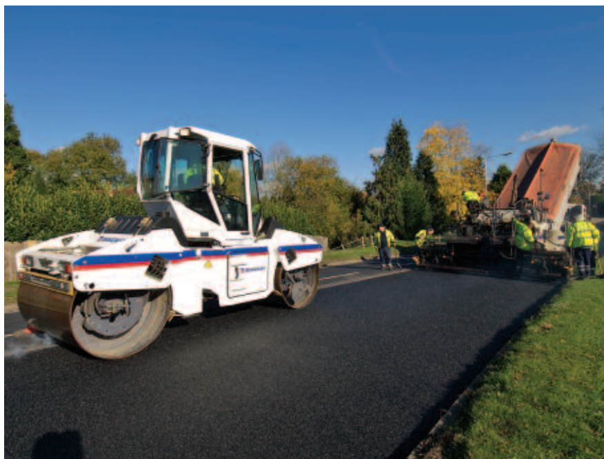
A roller compacts the Ultraphone surfacing to a depth of 60mm
