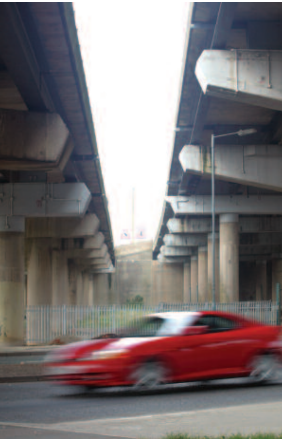
Ray Hall Viaduct on the M5/M6 junction was resurfaced and then reopened in one single overnight carriageway possession
