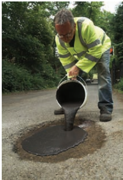
Pothole Filler is simple and quick to lay: (from left to right) preparation is minimal, application involves mixing and pouring the pre packed materials into the defect to form a durable and flexible repair which can be trafficked within 30 minutes.
