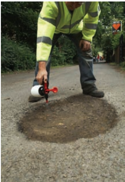
Pothole Filler is simple and quick to lay: (from left to right) preparation is minimal, application involves mixing and pouring the pre packed materials into the defect to form a durable and flexible repair which can be trafficked within 30 minutes.
