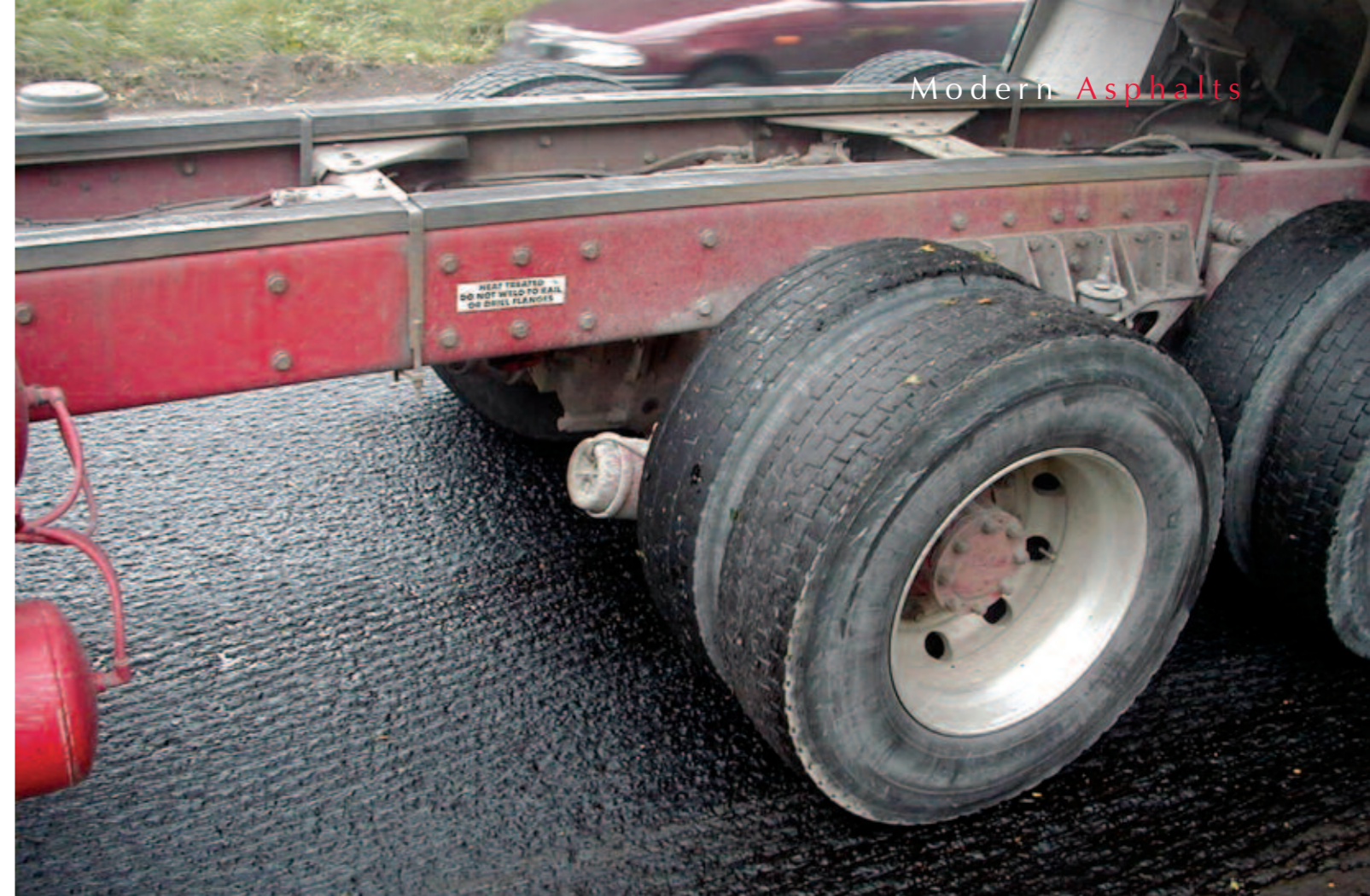
Nynas’ non pick up bond coats do not stick to tyres and remain inert until they receive asphalt
