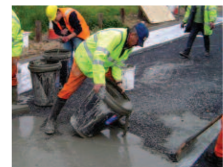
Flexicrete is laid swiftly in a two-stage process
