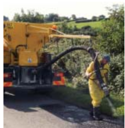
The Jetpatcher system is based on the technology of velocity patching
