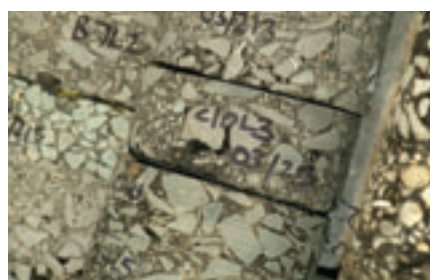
Asphalt testing is a key aspect of SWPE's expertise.
