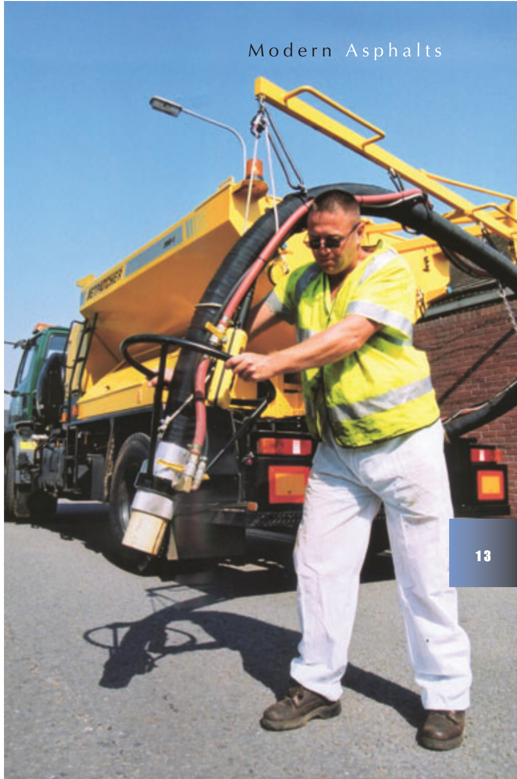
Use of Jetpatcher to repair potholes has helped several local authorities cut accident claims.
