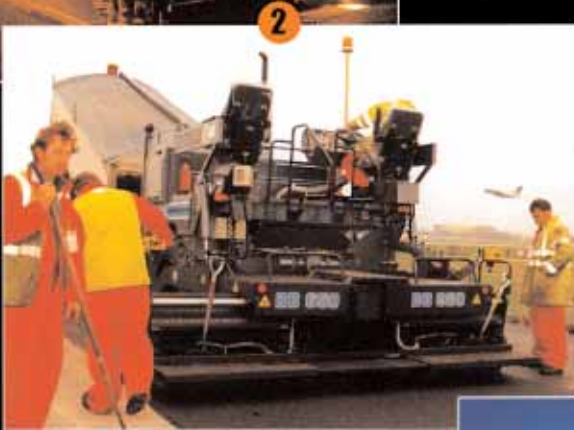
1. Thin surfacings such as Hanson's Tuffgrip can be laid quickly to provide a durable surface
