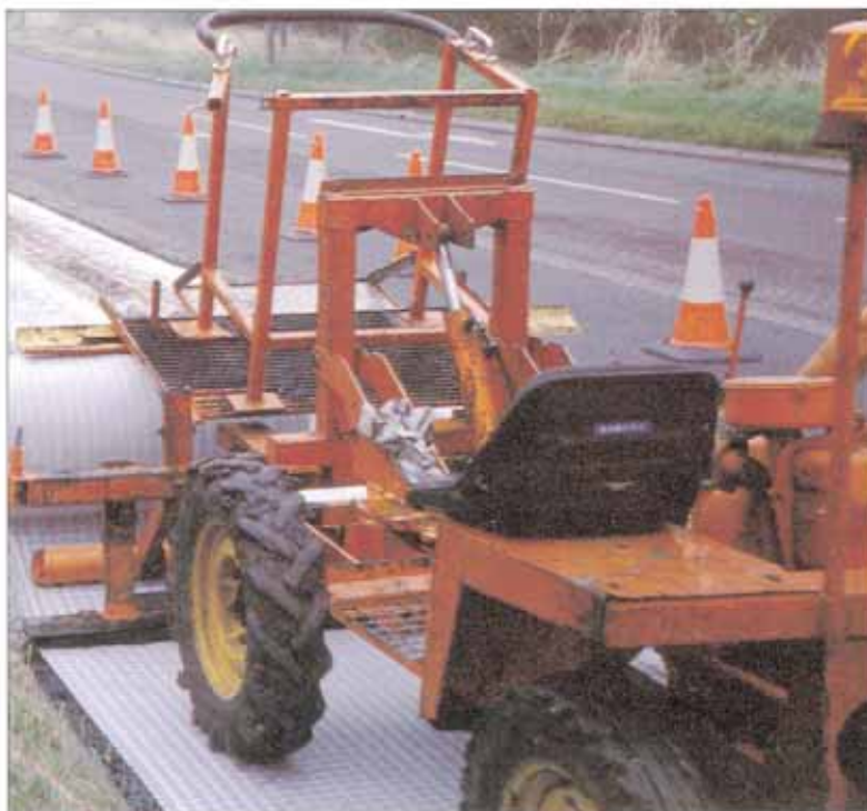
Laying Mastergrid to control reflective cracking through surfacing.
