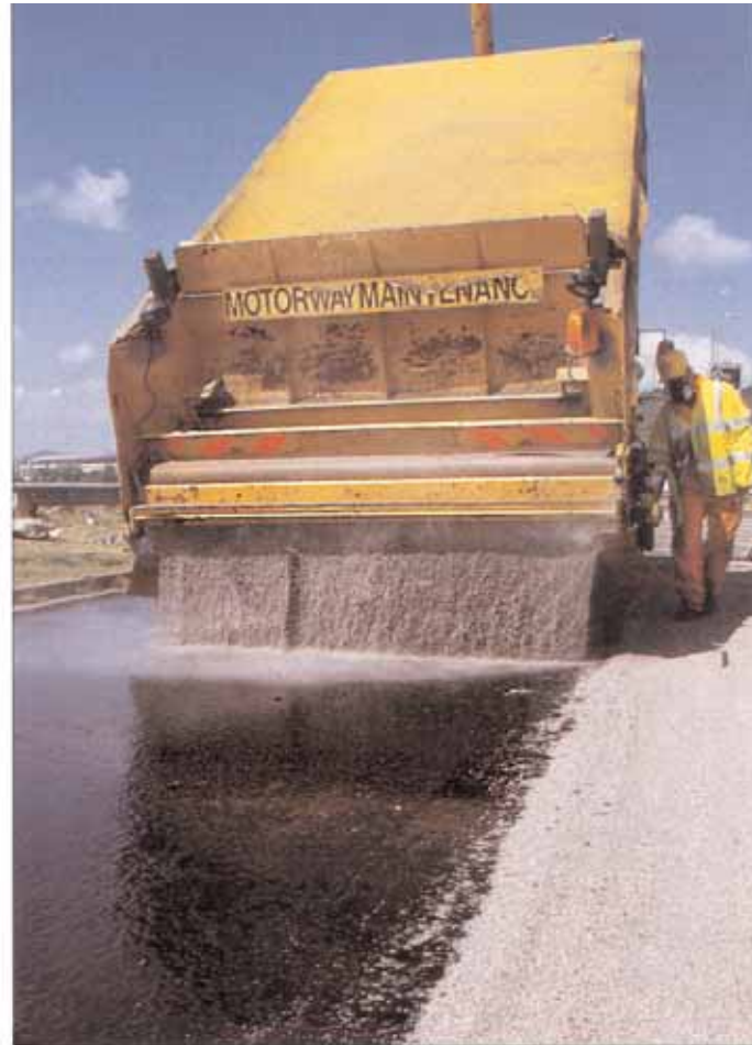
Anti skid surfacing Mastergrid being applied at a high stress site.
