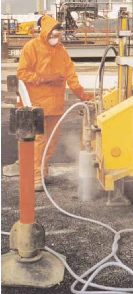
Cores prove that Foamix strengthens over its lifetime.
