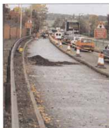
The A332 at Bagshot – before and after Foamix reconstruction.
