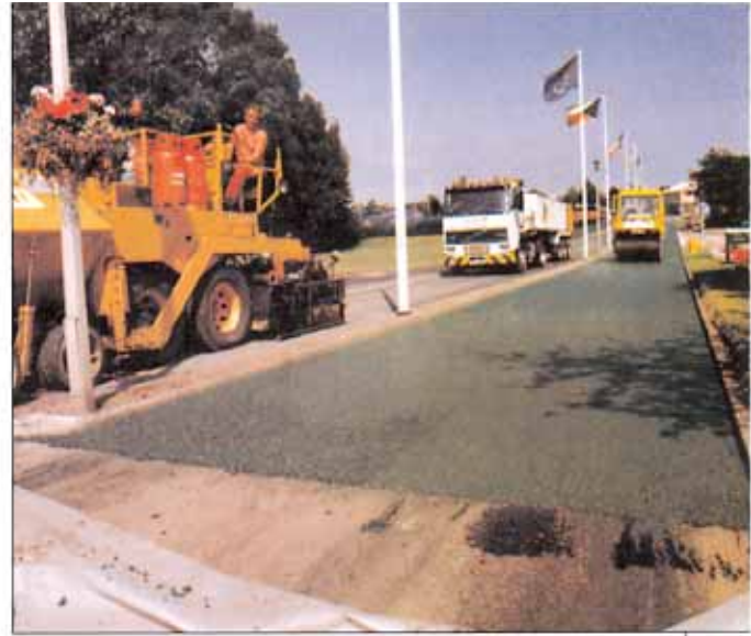
above: Laying Mastertint at TQP's headquarters left: Cycle routes can be clearly delineated using coloured asphalt far left: Masterprint targets the block paving market
