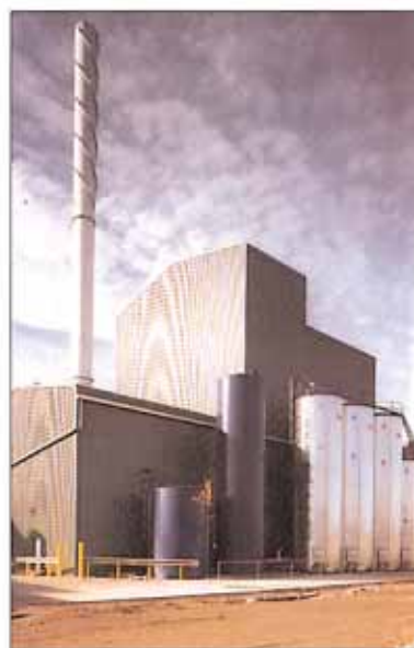
Crawley is Foster Yeoman's ideal of what an urban asphalt plant should be
