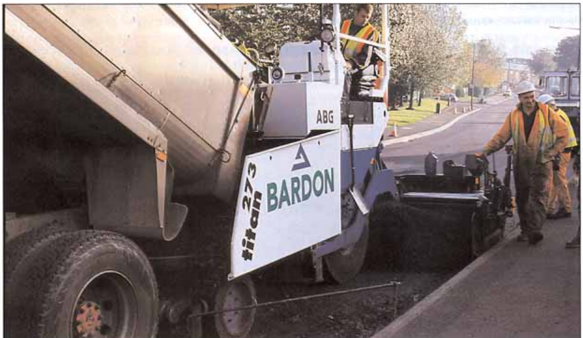
ASHphalt being laid in Dudley
