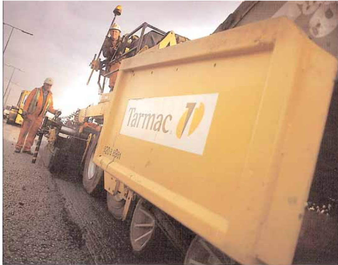
Planing old carriageway with hightech recycling in mind
