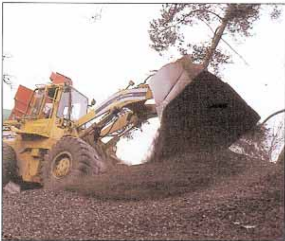
Stockpiling recycled material
