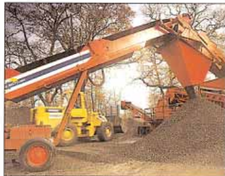
Crushed materials are screened to match a grading envelope
