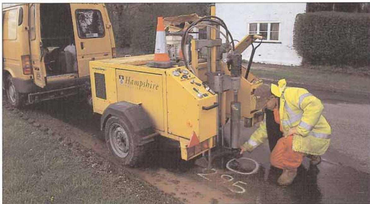
Extensive testing of Bardon's pioneering coldlay materials has proved their worth
