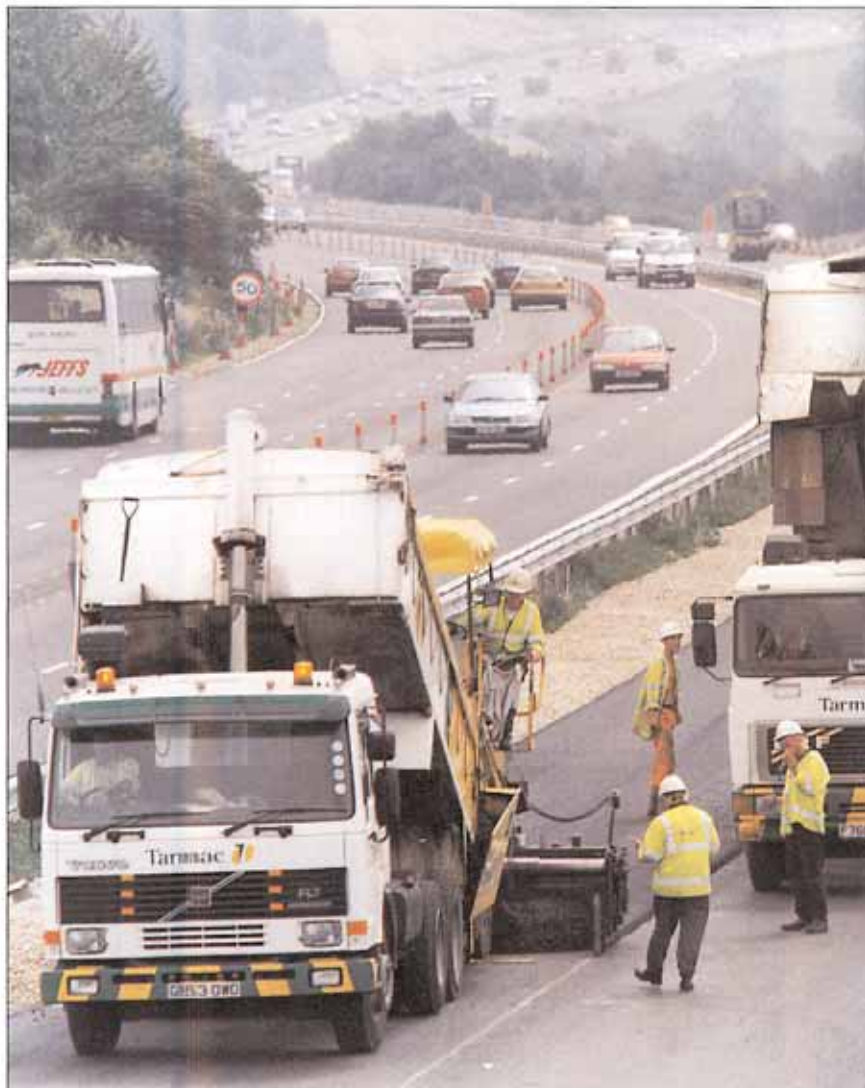
Tarmac laying Masterpave in echelon on the M40 near Oxford.
