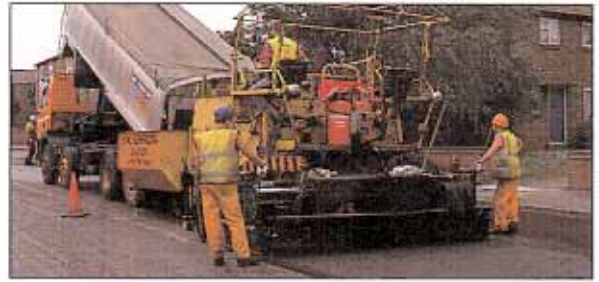
RMC Surfacing operatives doing a good job.
