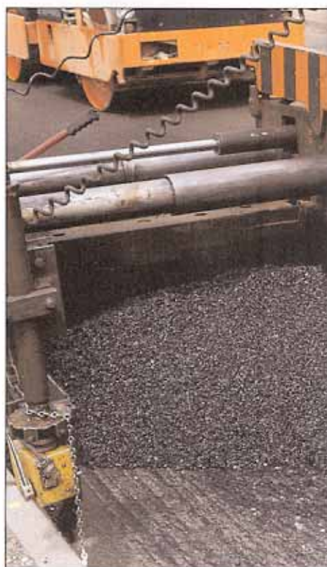
Viatex being laid to form a durable, safe sur-
