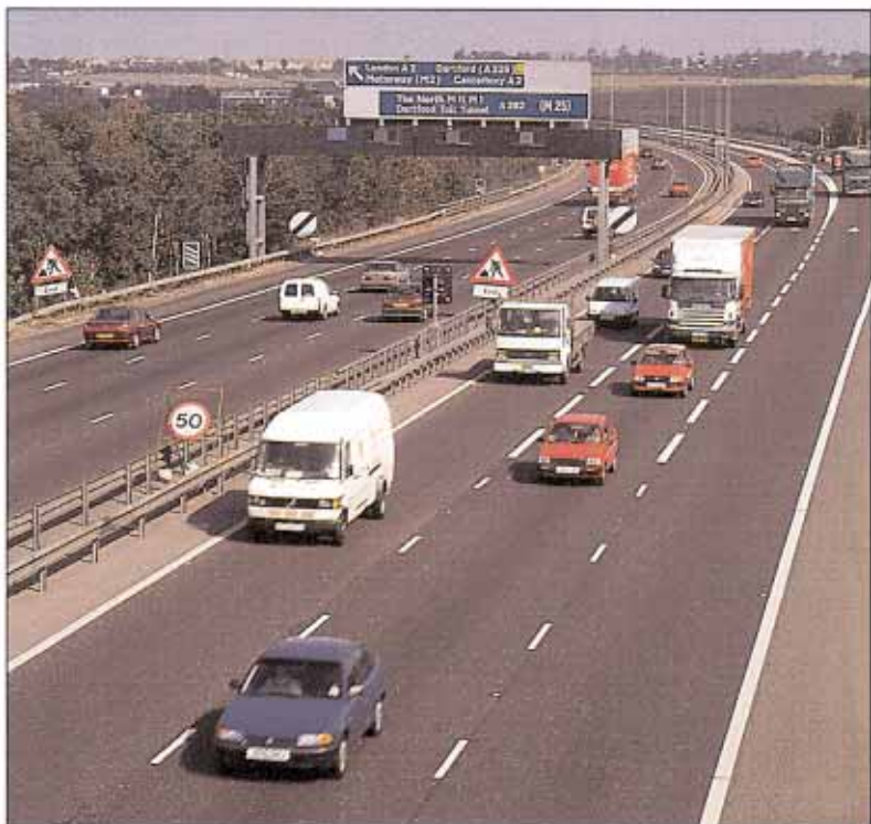
Long life pavements are likely to be whole life cost effective.
