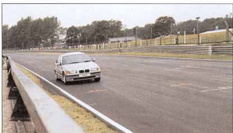
Benefits of the advanced asphalt surfacings used recently at Brands Hatch and Silverstone are also available for public highways. The transfer of asphalt technology from the race track to roads confers advantages of durability and skid resistance while offering smoother, quieter and safer roads for the motorist. These modern asphalts developed by companies appearing in this magazine display all the characteristics needed to meet the demands of today's heavily trafficked roads.
