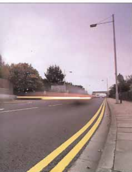
urfacing for fast moving urban traffic.
